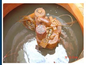
The picture to the left is of a product piping submersible pump with *Secondary Containment*. It is designed to capture any spilled or leaked petroleum from your storage tank system, whether it is from the tank or piping. Containment can be located around the tank or at various locations within the piping system, such as tank-top, transition, and under dispenser. In order to benefit from secondary containment, it must be maintained.
